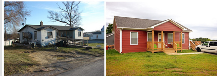
BEFORE & AFTER of a substantial reconstruction in the Baskerville Neighborhood
