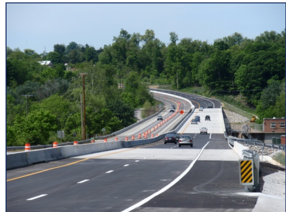
Route 114 Bridge Completed 2014
