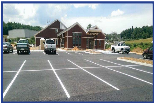
The Floyd Innovation Center will be completed in the fall of 2014 with the help of Economic Development Administration, Appalachian Regional Commission, and Tobacco Commission funding.
