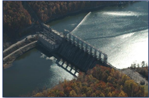
Claytor Lake Dam, Credit: Peter Huber
