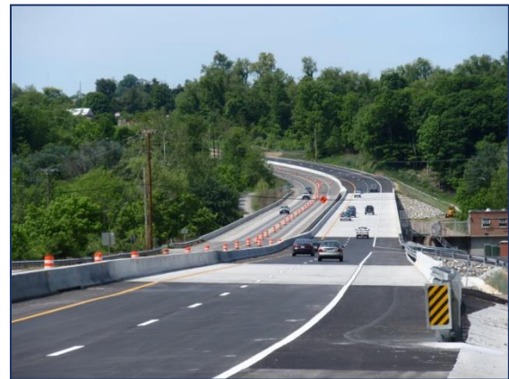
Route 114 Bridge Completed 2014
