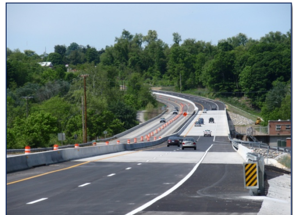
Route 114 Bridge Completed 2014
