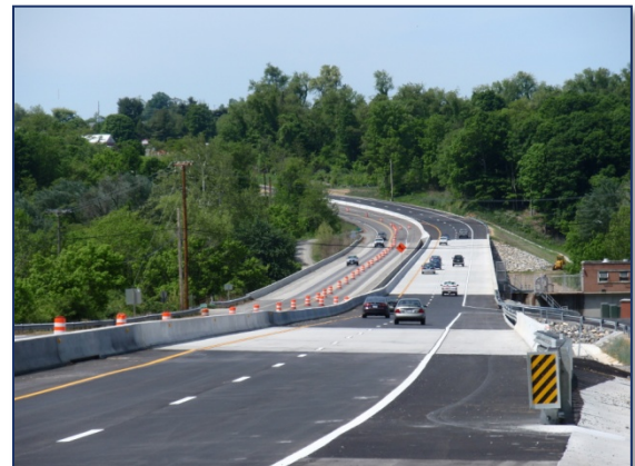
Route 114 Bridge Completed 2014
