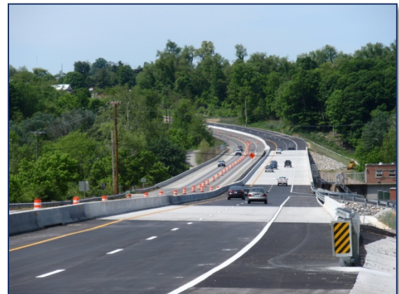
Route 114 Bridge Completed 2014
