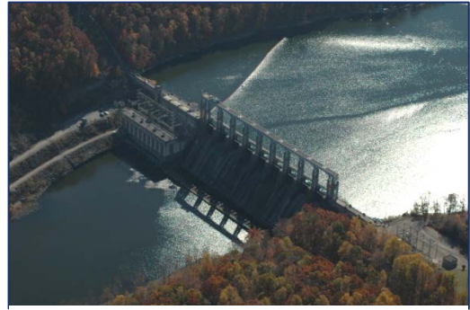
Claytor Lake Dam, Credit: Peter Huber
