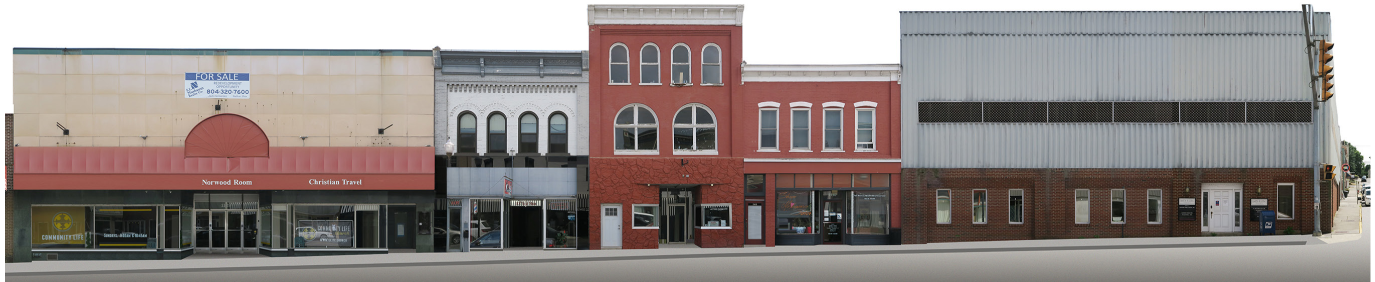
WEST END EXISTING STOREFRONT
