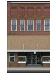
EXISTING STOREFRONT C
